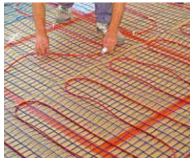
Heating cables connection.
