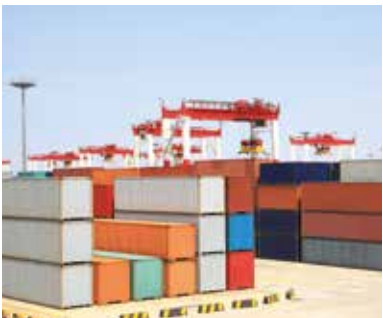
Wiring in shipbuilding and cooling containers.
