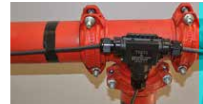
Connection of heating cables (France). Series TH211.
